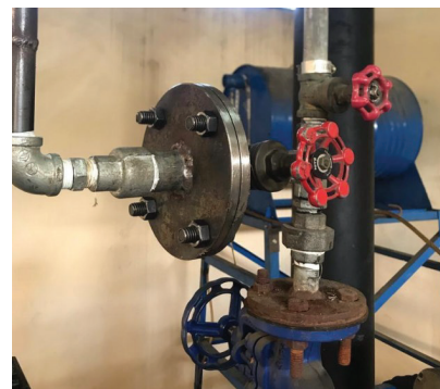
Fig. 3. Installation of the gasket on the flange in the boiler line
